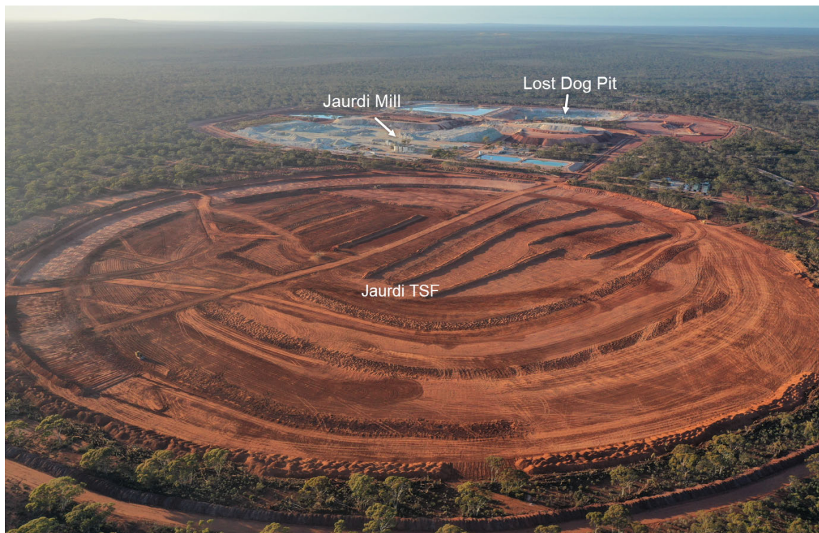
Figure 1: Jaurdi Tailings Storage Facility on 8 October 2021
