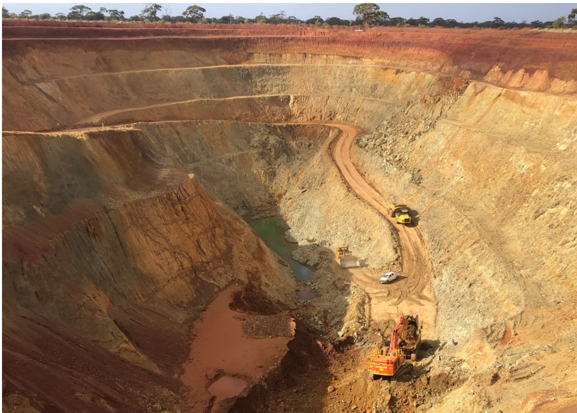
Figure 2: Looking south at the Panther Pit on 2 March 2021
