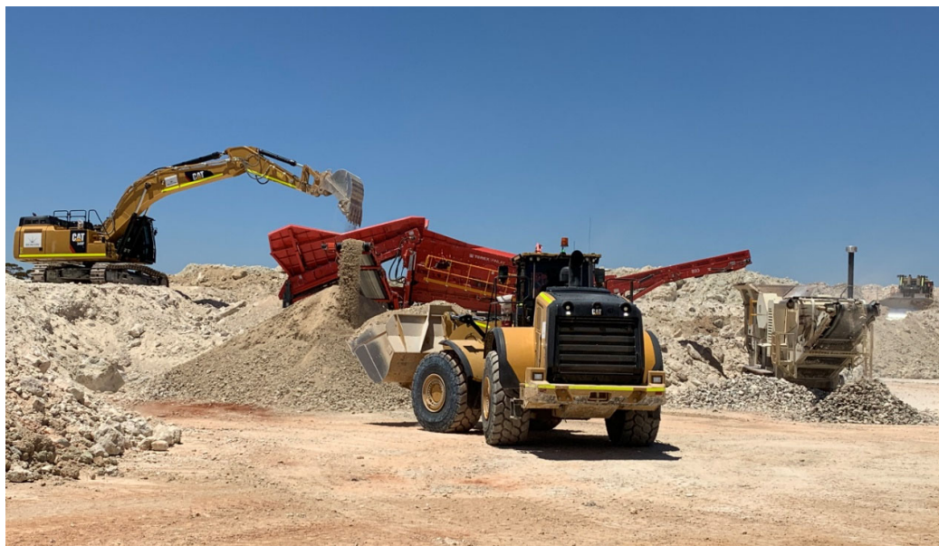
Figure 3 – Screening and Crushing on the Jaurdi ROM pad.
