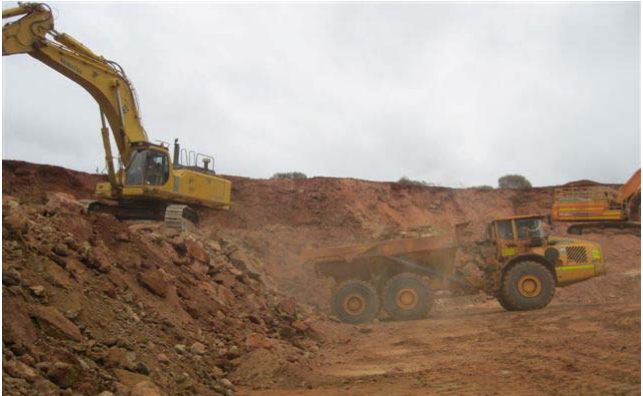
Top soil and overburden removal at Halleys East
