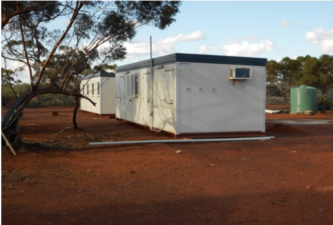
Accommodation Dongas included in the acquisition of the Halleys East camp
