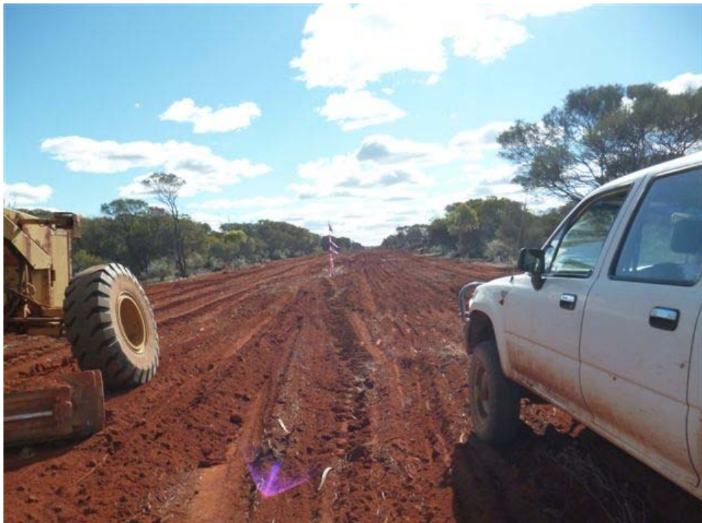
Construction of the haul road access to Halleys East being completed
