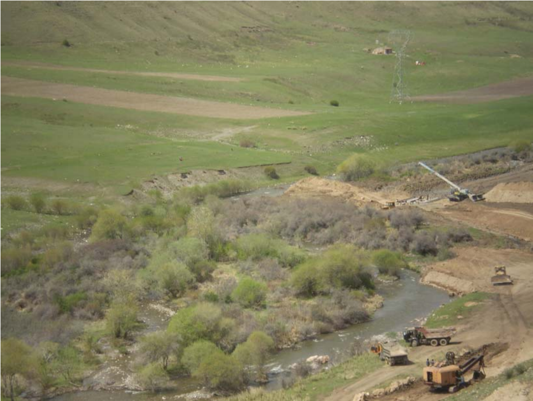
Attachment 6: Baladjan Silicon Project– Site Photos. Outcropping quartzite ridge at Baladjan (part of Area 1, above) & view looking from Quartzite ridge showing road, bridge construction and power lines
