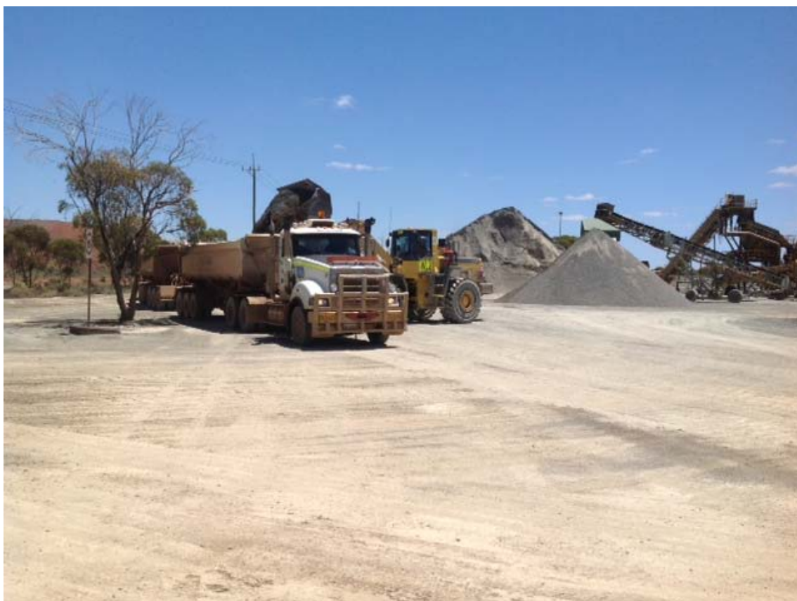
Figure 1 – Commencement of Crushing and Sampling - February 2016
