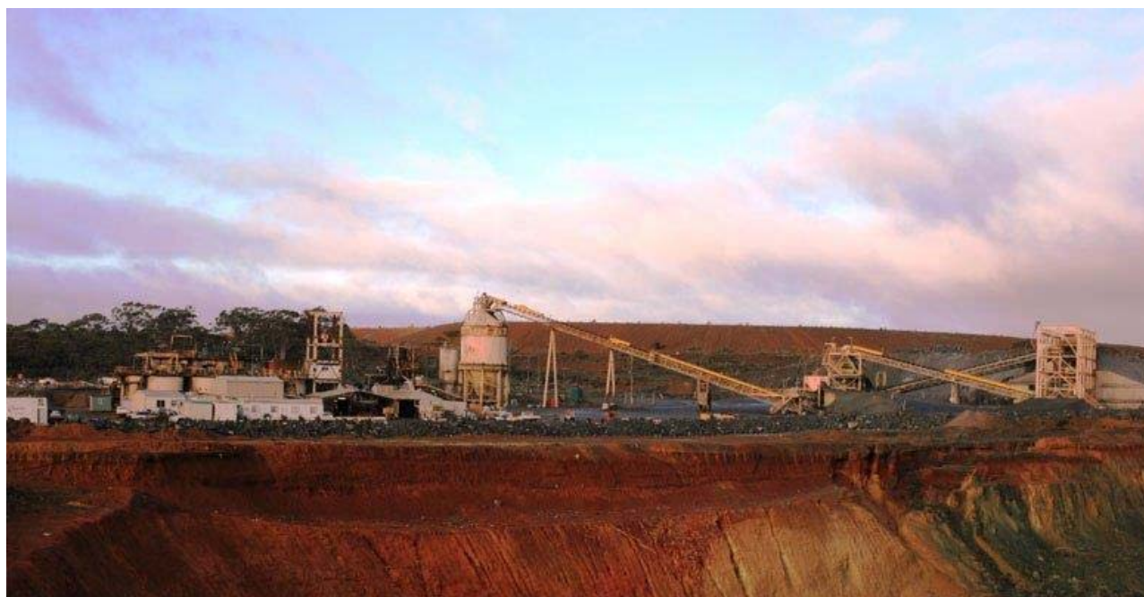
Figure 3: Greenfields Mill, Coolgardie Western Australia
