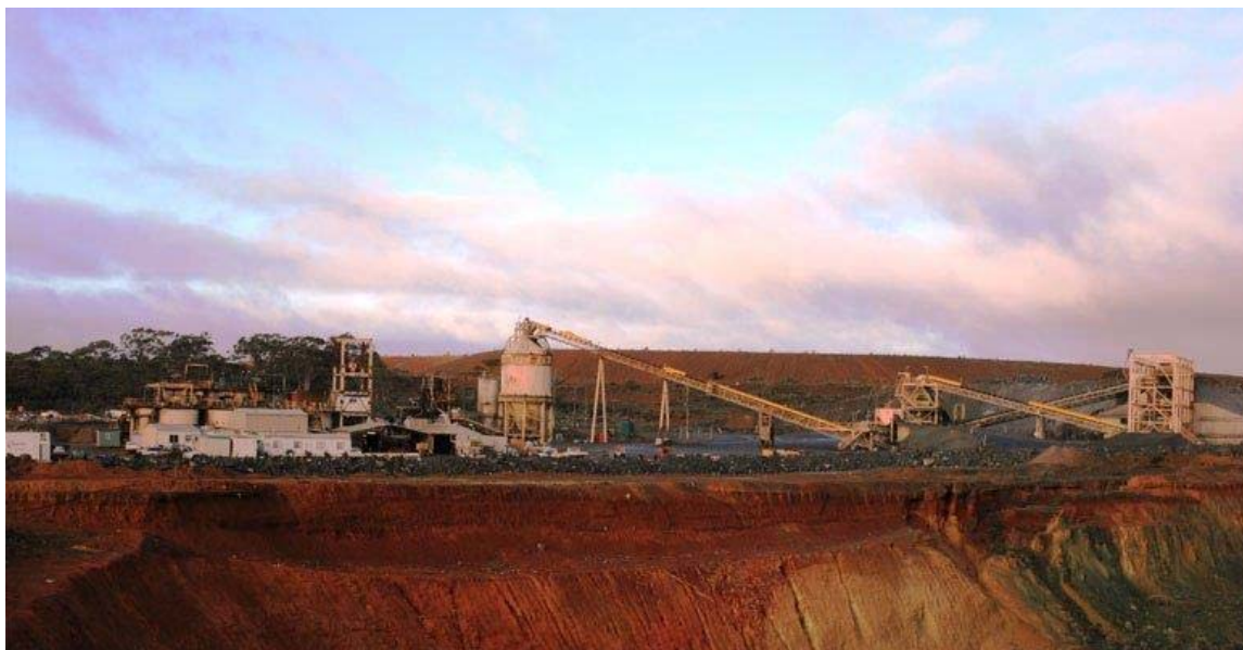
Greenfields Mill, Coolgardie Western Australia
