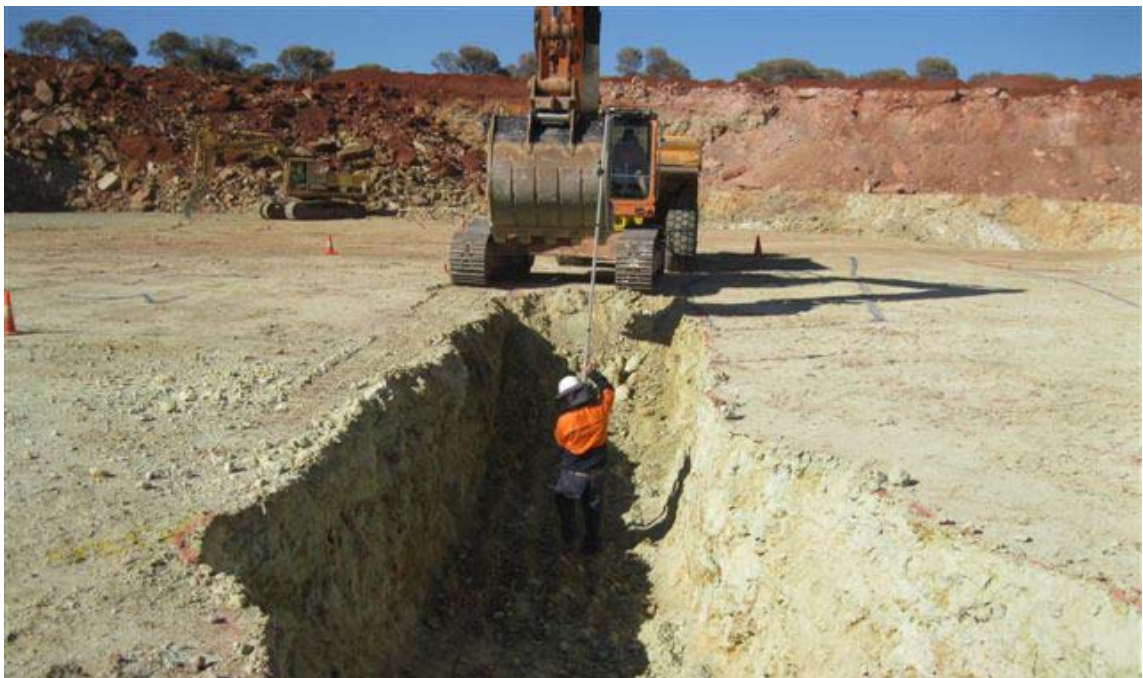
Ore being selectively mined at Halleys East
