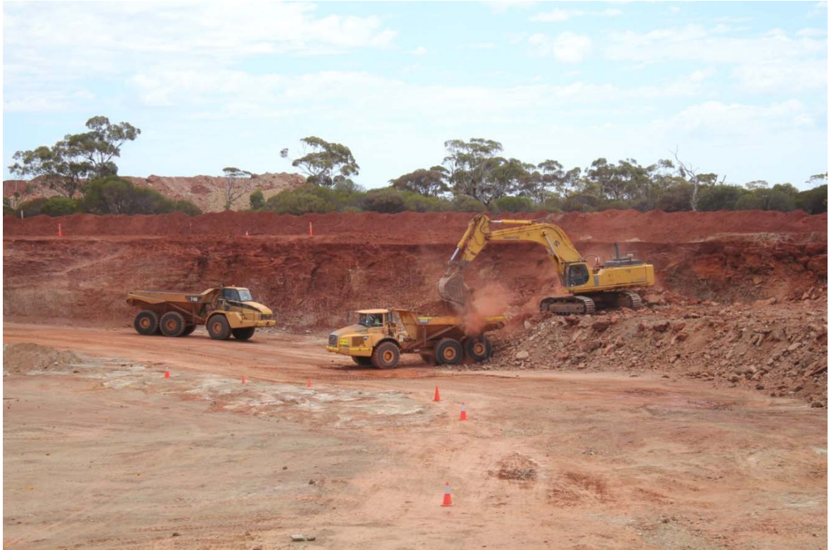
Removal of waste at the Halleys East open pit
