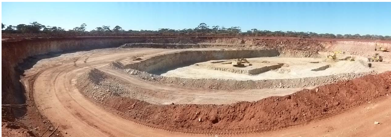
Halleys East open cut mine 16 January 2014
