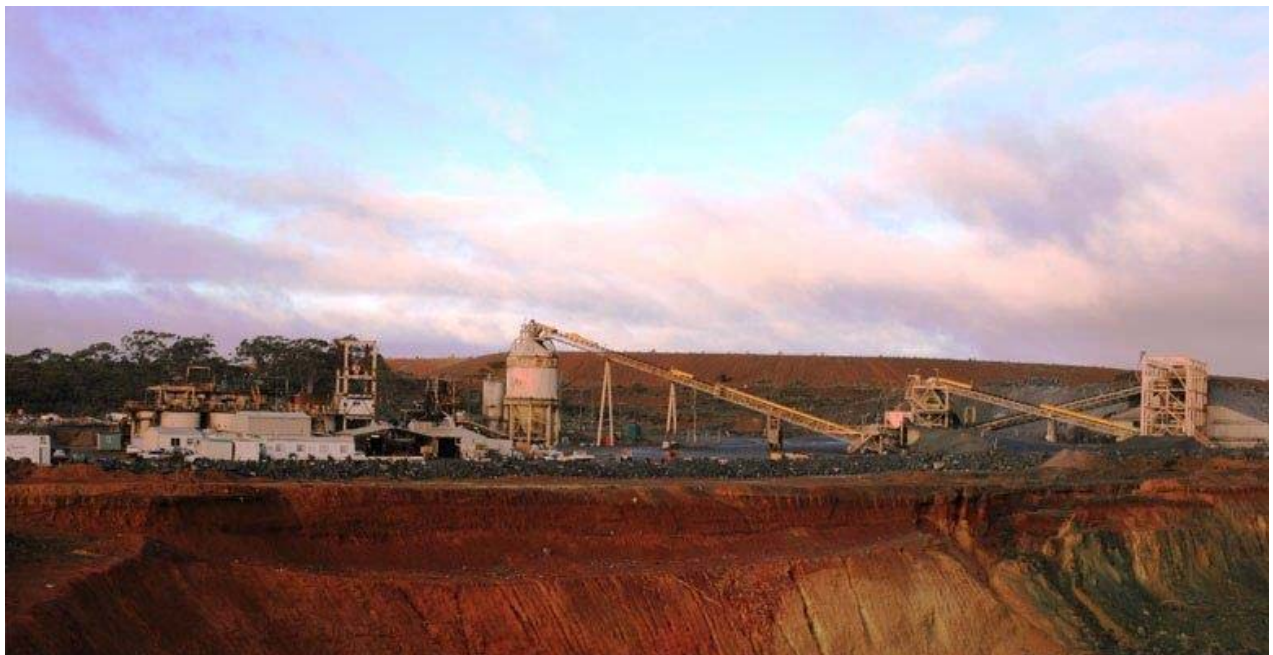
Greenfields Mill, Coolgardie Western Australia
