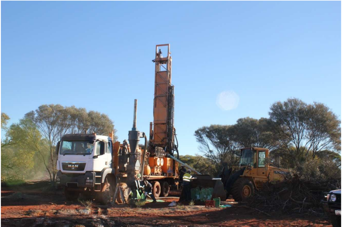
Percussion Drill Rig In Operation at Halleys East
