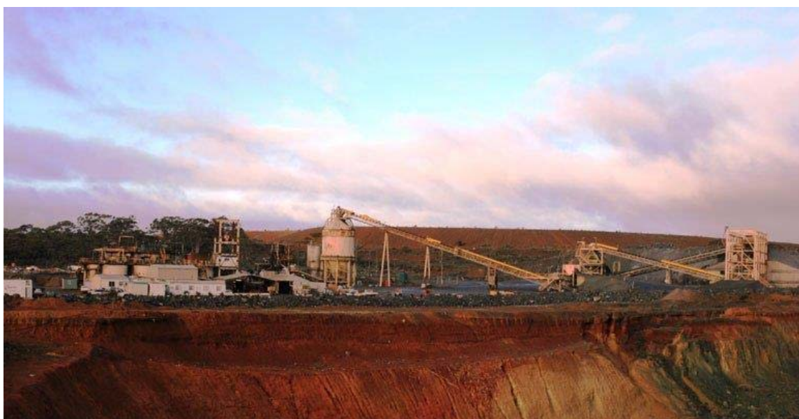
Greenfields Mill, Coolgardie Western Australia
