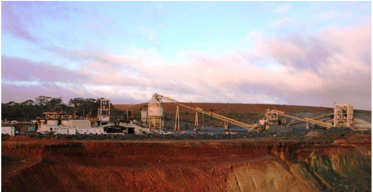
Greenfields Mill, Coolgardie Western Australia
