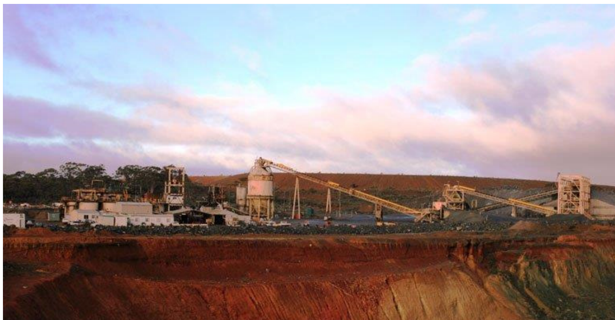
Greenfields Mill, Coolgardie Western Australia
